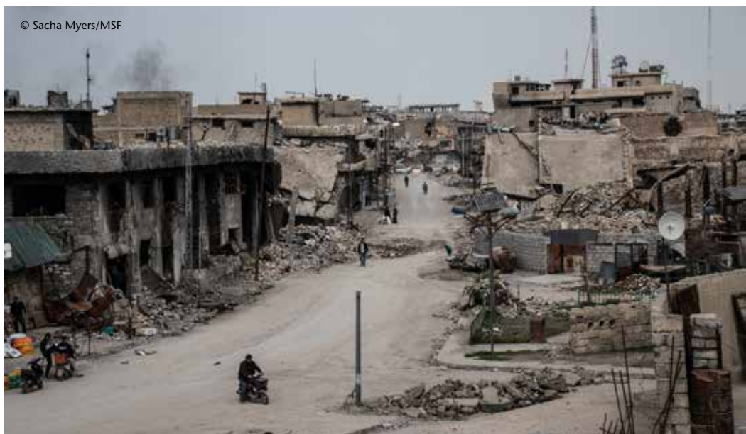
The Old City in Mosul, pictured in April 2018, when much of the city remained inaccessible due to the destruction and presence of improvised explosive devices, unexploded ordnance and booby traps.
