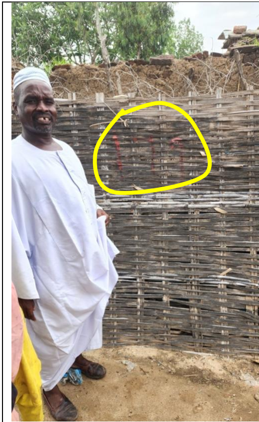
Plate 5a: Rehabilitated latrine in Kass
