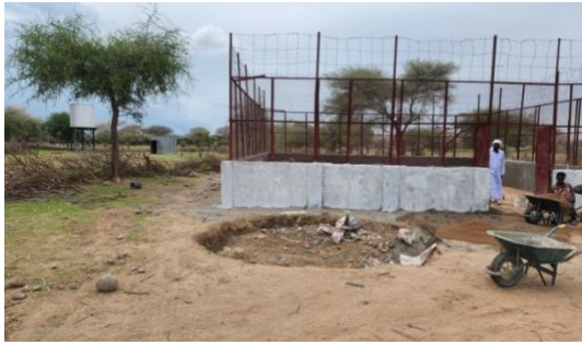
Plate 9c: Jabra WY under construction
