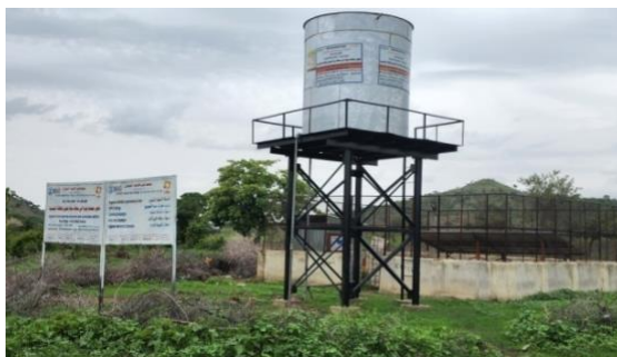
Plate 9a: Rehabilitated WY at Fiena village
