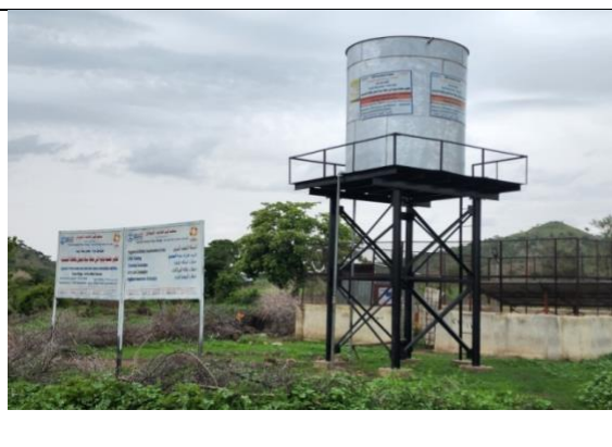
Plate 8b: Water facility in Fiena supported hybrid system.
