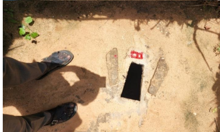
Plate 5b: Constructed latrine at Elsalam
