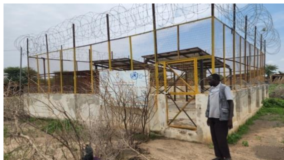
Plate 9b: WY supported by solar system in Kass
