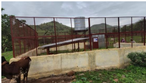
Plate 8d: Existing HWY supported at Fiena village
