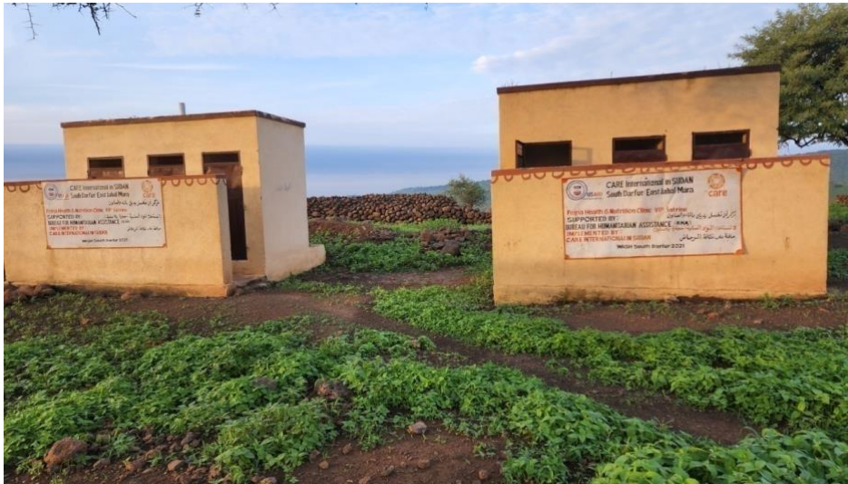
Plate 9e: Males and females latrines constructed at Fienna H & N center.
