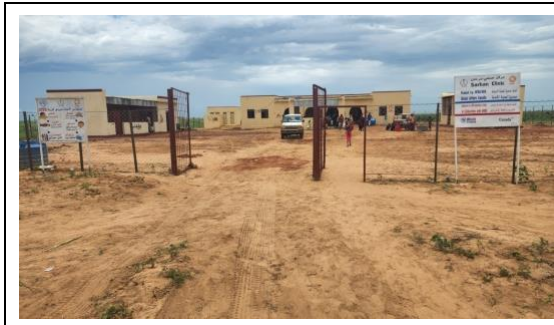
Plate 9j: Surhan health and nutrition centers, under construction
